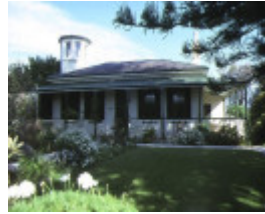
1 roseville cottage mercer street queenscliff front view
