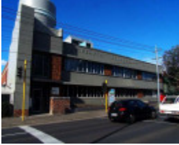
RICHMOND HODDLE STREET 129
