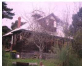
1 ballara glaneuse road point lonsdale rear elevation jun1995
