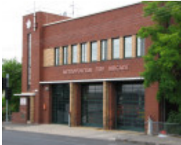
BRUNSWICK FIRE STATION AND FLATS SOHE 2008
