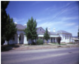
alexandra court house & shire hall street view feb1985
