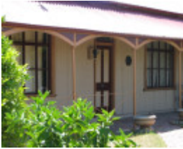
IRON HOUSE SOHE 2008
