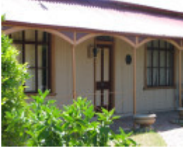
IRON HOUSE SOHE 2008
