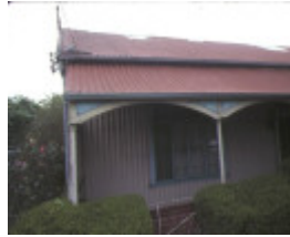
1 iron house brunswick road brunswick front view aug1980
