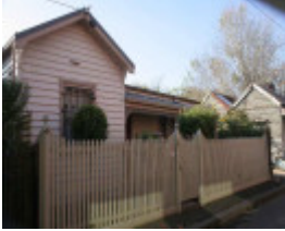
RICHMOND SHAMROCK STREET 5.jpg
