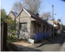
RICHMOND SHAMROCK STREET 7.jpg
