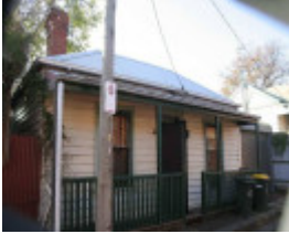
RICHMOND SHAMROCK STREET 9.jpg
