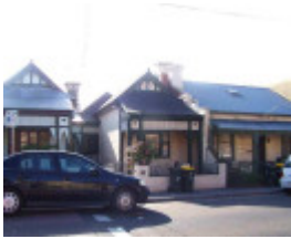
RICHMOND BAKER STREET 55.jpg
