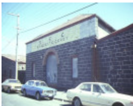
former melvilles grainstore colebrook street brunswick entrance
