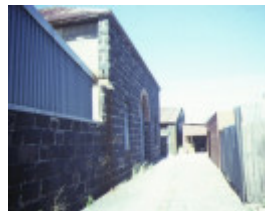
former melvilles grainstore colebrook street brunswick rear of buildings 3 & 4
