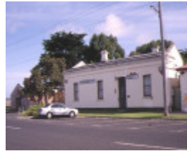
1 bond store & office port albert front view feb 1996
