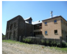
FORMER COBB & CO STAGING STABLES SOHE 2008
