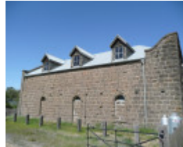
FORMER COBB & CO STAGING STABLES SOHE 2008
