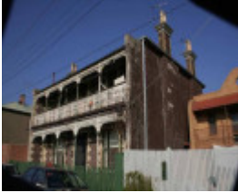
Richmond LESNEY STREET 20.jpg
