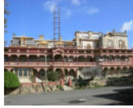
Eastern elevation of the house .jpg
