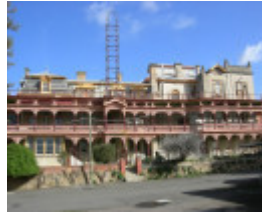
Fortuna_Bendigo_east elevation_3 August 2009
