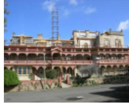
Eastern elevation of the house .jpg
