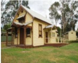
FORMER HEALESVILLE COURT HOUSE SOHE 2008
