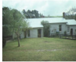
former state school number 46 school lane bulla side elevation aug1985
