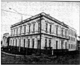
Ballarat City Council Offices - Ballarat Heritage Review, 1998
