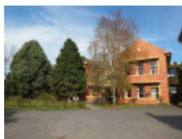
North elevation, Fatima House (Building 10)
