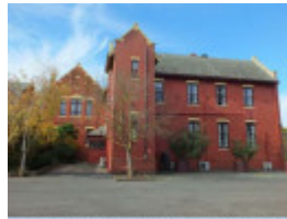
West elevation, Orphanage Additions (Building 5)
