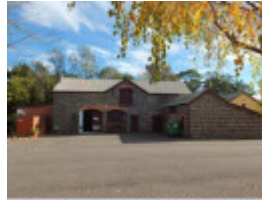
East elevation, Stables & Machinery Shed (Building 2)
