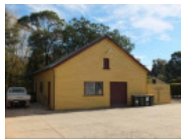
East elevation, Galined Shed (Building 8)
