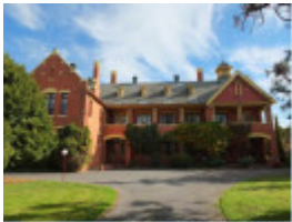
East elevation, St Joseph's Orphanage (Building 3)
