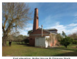
East elevation, Boiler House & Chimney Stack (Building 11)
