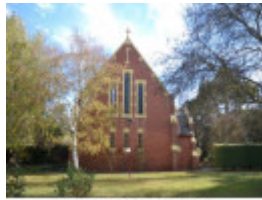
East elevation, Chapel (Building 4)
