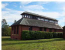
South & east elevations, former Laundry (Building 7)
