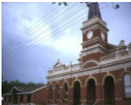
buninyong town hall street frontage dec1987
