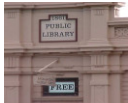
former library buninyong signage detail 2002
