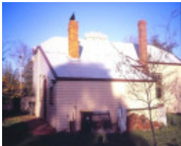
former library warrenheip road buninyong rear view she project 2003
