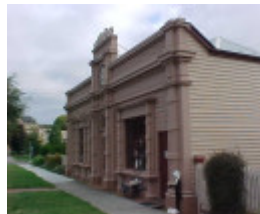
former library buninyong oblique front view 2002
