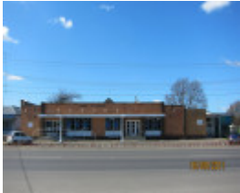
Sebastopol Town Hall complex - 1960 Borough Hall
