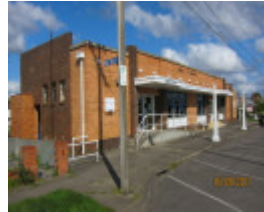
Sebastopol Town Hall complex - 1960 Borough Hall
