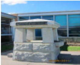
Sebastopol Town Hall complex - King George V Memorial drinking fountain
