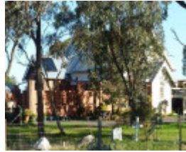
former St Francis Xavier Catholic Church, east elevation with red brick addition
