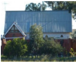
former St Francis Xavier Catholic Church, east elevation from the Loddon Valley Highway
