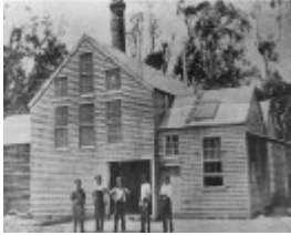
John Goyne's factory (demolished)
