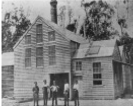
John Goyne's factory (demolished)
