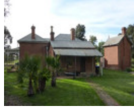
South elevation of Rosemundy House, with the scullery, c.1858 at centre, the 'gold office' at right and the west wing, c. 1890s, at left.
