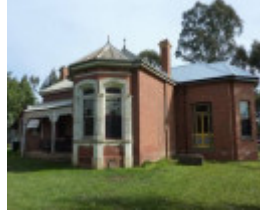
East elevation, the verandahed component at left dates to c. 1867, the faceted bay window to the 1890s and the north wing, at right, to 2007.
