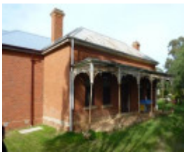
West elevation, 1890s.
