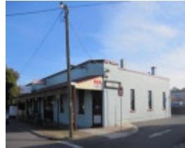
South and east elevations (2010).
