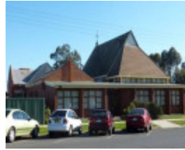
Rear (east) of the Uniting Church complex.
