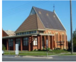
East elevation. The addition was built in 1986 following a fire.
