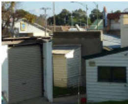
Rear of the property (centre of image).
