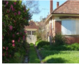
Motor garage to the north of the house.
