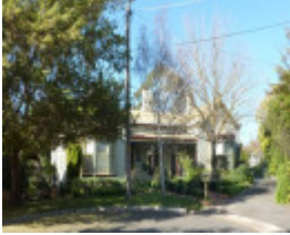
West elevation of Myrnong.
