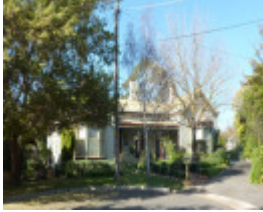
West elevation of Myrnong.
