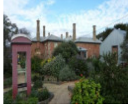
West elevation, viewed from Morrison Street.
