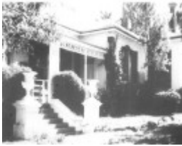
Front (north) elevation, c. early 1990s (Source: Photographic History of Kangaroo Flat, 1994, v. 1).
