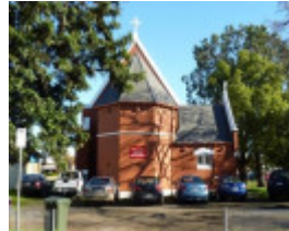
Rear (east) view, with sanctuary at centre and sacristy to the right.
