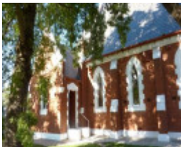
Entry to the sacristy (north elevation).
