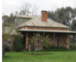
South-east elevation, note timber dormer at rear.
