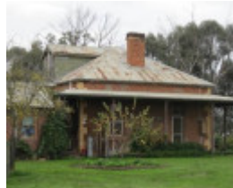
South-east elevation, note timber dormer at rear.
