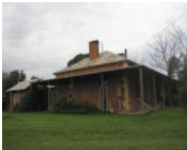
View of Ark Hall looking directly east.
