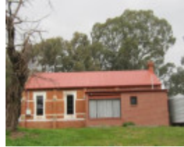
North elevation, with recent addition.
