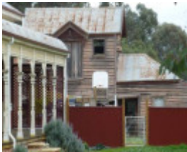
East elevation of the stables, with the verandah of the presbytery at right.
