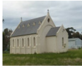
St Patrick's, north and west elevations.
