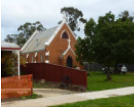
East elevation of the former Holy Trinity Anglican Church, Marong.
