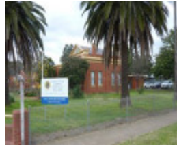
West elevation, note mature palms.
