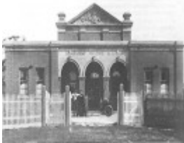
Shire of Marong Hall c. 1908 (Source: Mike Butcher and Gill Flanders, Bendigo Historic Buildings, National Trust of Australia. p. 167).
