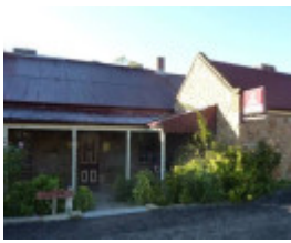
Former residence, to south of 1865 wing.
