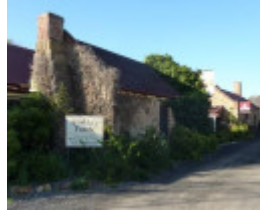
The 1860s wing; note stepped chimney form.
