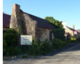
The 1860s wing; note stepped chimney form.
