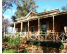
North elevation, note recent verandah.
