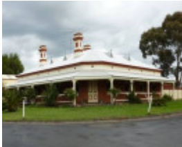
View of the present Shamrock Hotel from the north-east. Note chimneys.
