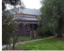
Verandah at west of property.
