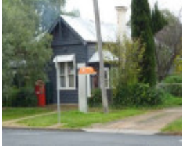
Post office entrance, at east of property.
