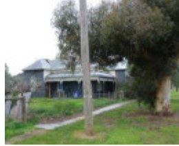
West elevation, as viewed from Inglewood Street.
