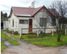
South elevation. Note infilled verandah to the west of the projecting gable.
