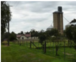
East elevation, with grain silo at rear.
