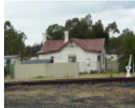
West elevation, with the rail track in the foreground.
