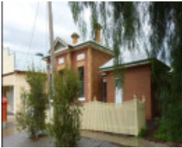
View looking north-east; note west addition at right.
