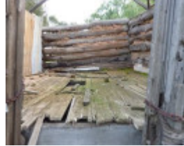
Raised floor and remnant mud and brick pugging to the eastern store
