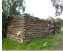
View of site from Rothackers Road (west)
