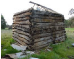
The eastern store, viewed from the south-west
