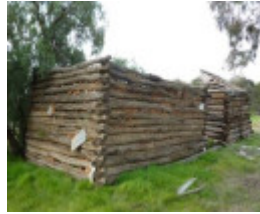
View of site from Rothackers Road (west)
