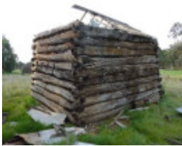
The eastern store, viewed from the south-west
