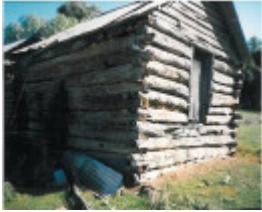
East end of eastern store
