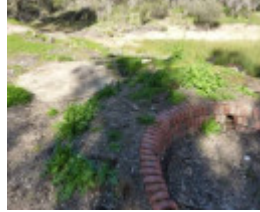
Brick vats adjacent to the stack.
