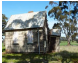
West elevation, note partially detached entrance porch.
