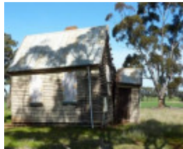
West elevation, note partially detached entrance porch.
