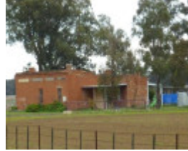
Former Royal Hotel, rear (east)
