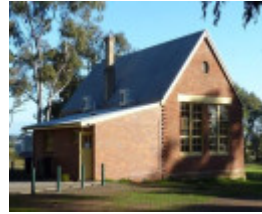
Woodvale Hall, rear (south) and east elevations, note skillion addition at left of picture
