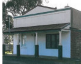
Former Old House at Home Hotel, pictured in August 2008
