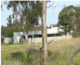
Former Old House at Home Hotel, north elevation, viewed from Camp Road
