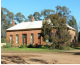
Former Camp Hotel and Store, east elevation
