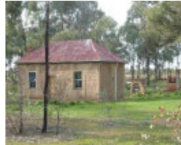
Kelly Cottage, west and south elevation of the cottage, note ruins of former kitchen at rear
