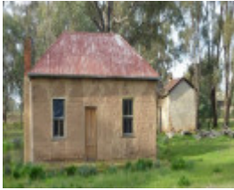
Kelly Cottage, front (west) elevation, with gable roofed outbuilding at right (south)
