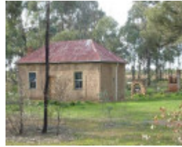
Kelly Cottage, west and south elevation of the cottage, note ruins of former kitchen at rear
